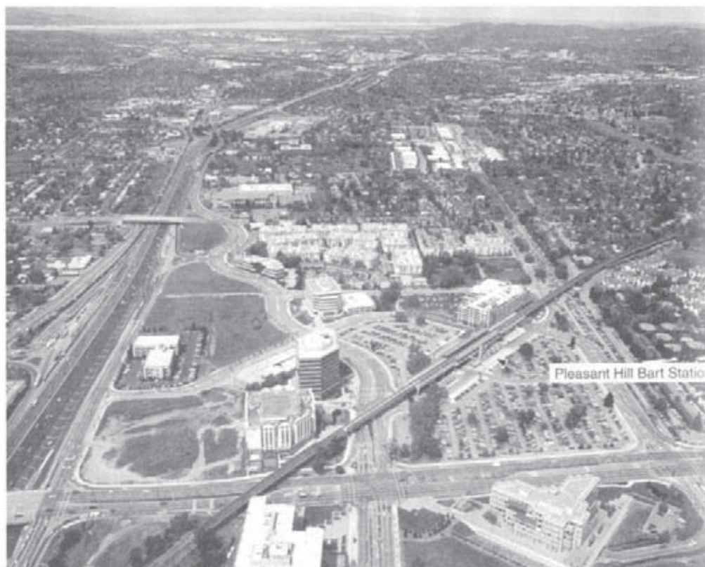
Fig. 11. Emergence of a transit village: Pleasant Hill Station, San Francisco, CA. 1994. The low-density coverage in the countryside is maintained, with new development concentrated at the transit station.
